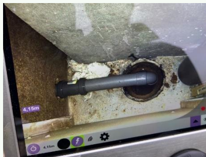
Missing vertical riser pipe, alternative pipe for kitchen drain created
